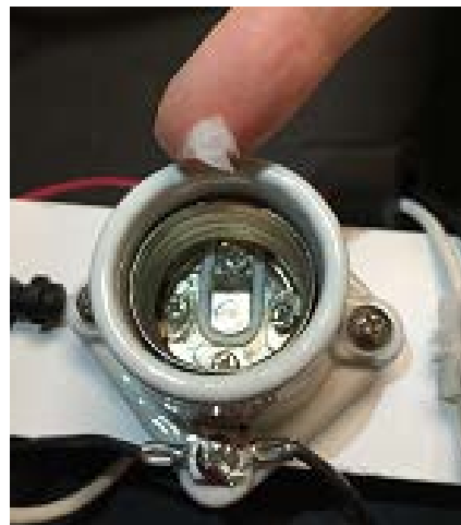
Figure 2, adding dielectric grease to sockets
