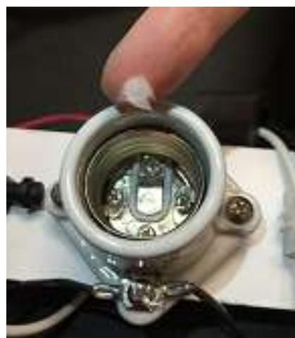
Figure 2, adding dielectric grease to sockets
