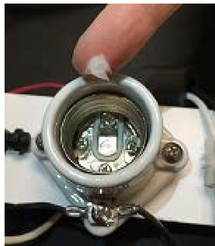
Figure 2, adding dielectric grease to sockets
