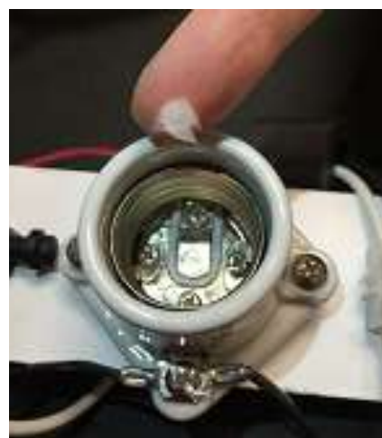
Figure 2, adding dielectric grease to sockets
